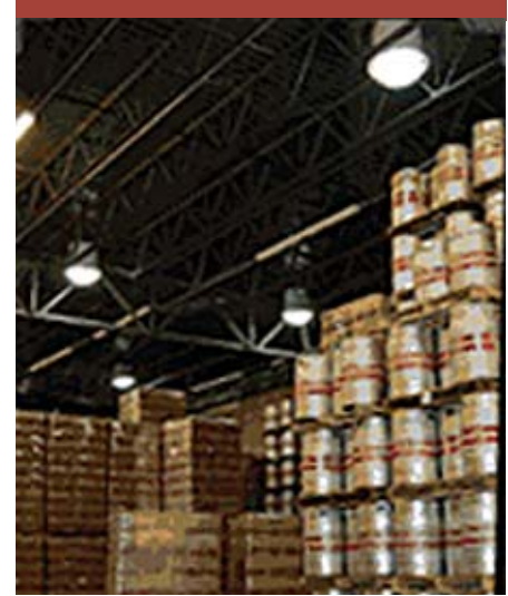
Light tubes provide natural lighting in the warehouse.
